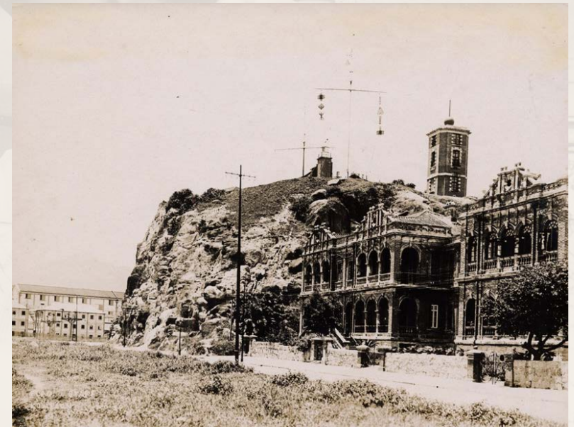
Figure 27: In the 1920s, the Observatory hoisted the China Seas Storm Signal Code (Non-Local Signals) at Signal Hill to deliver tropical cyclone information to ships in the harbour. (Photo courtesy of Mr. Shun Chi-ming, former Director of the Hong Kong Observatory)
